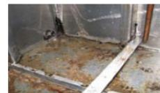
Figure 2 Corrosion Damage
