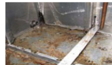
Figure 1 Corrosion Damage
